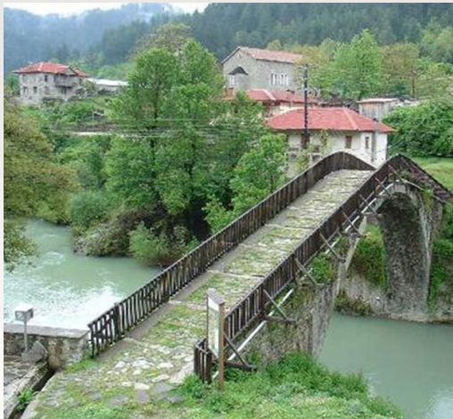
Bridge over Aaos River
